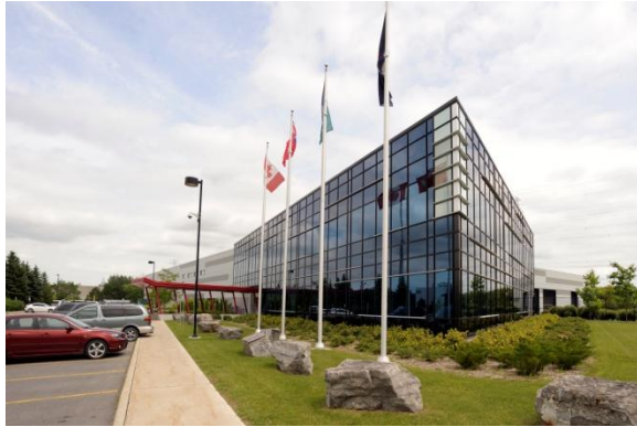
LEED Ambulance Station
