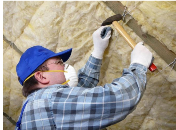
Home insulation installation
