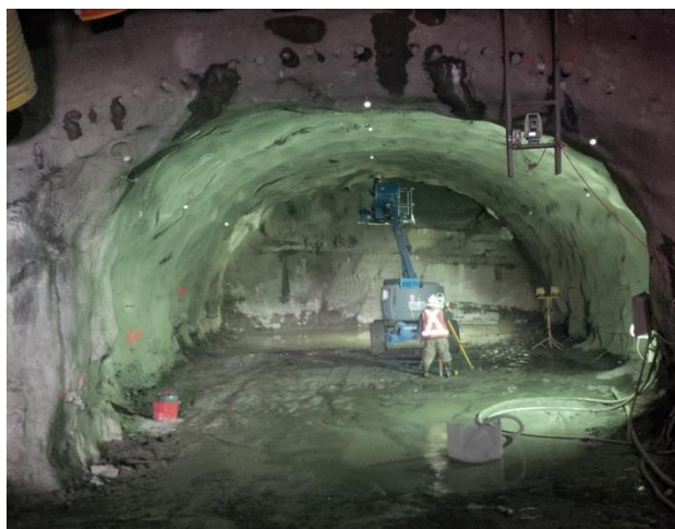
Light Rail Transit Tunnel Construction
