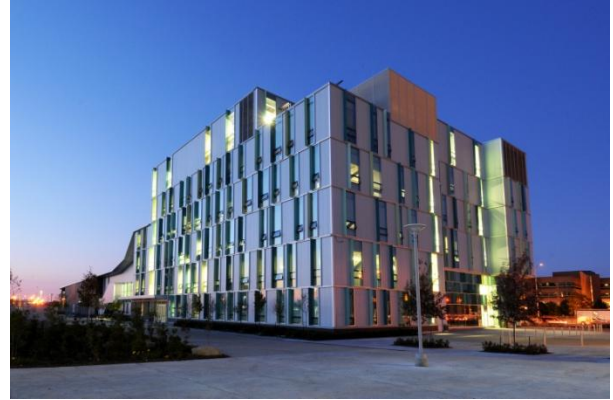
The Algonquin Centre for Construction Excellence at Algonquin College
