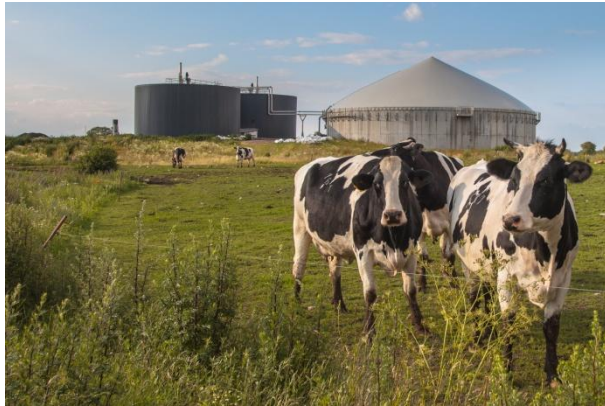
Agricultural Biogeneration Facility
