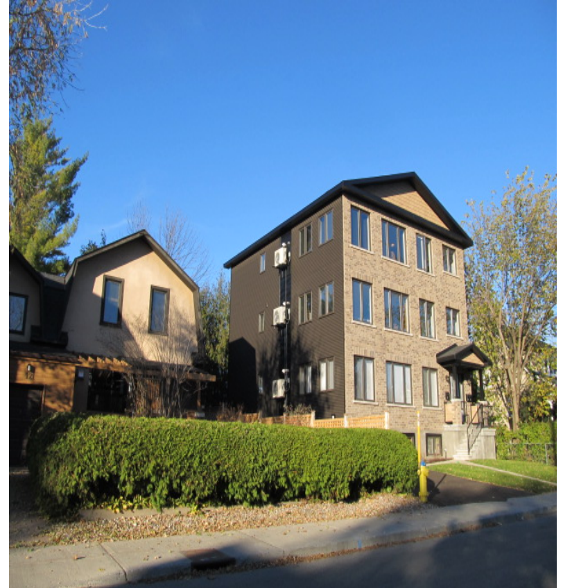
R3 Triplex converted to 4 plex. Streetscape issue.
