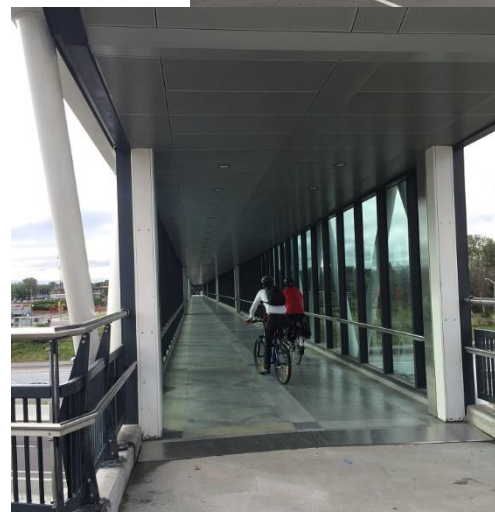
Bridge linking baseball stadium to Via Rail Station is excellent cycling infrastructure
